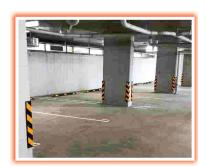
Application : Provide protection against damages caused by vehicles
